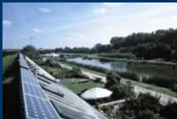
Hockerton earth-sheltered development
